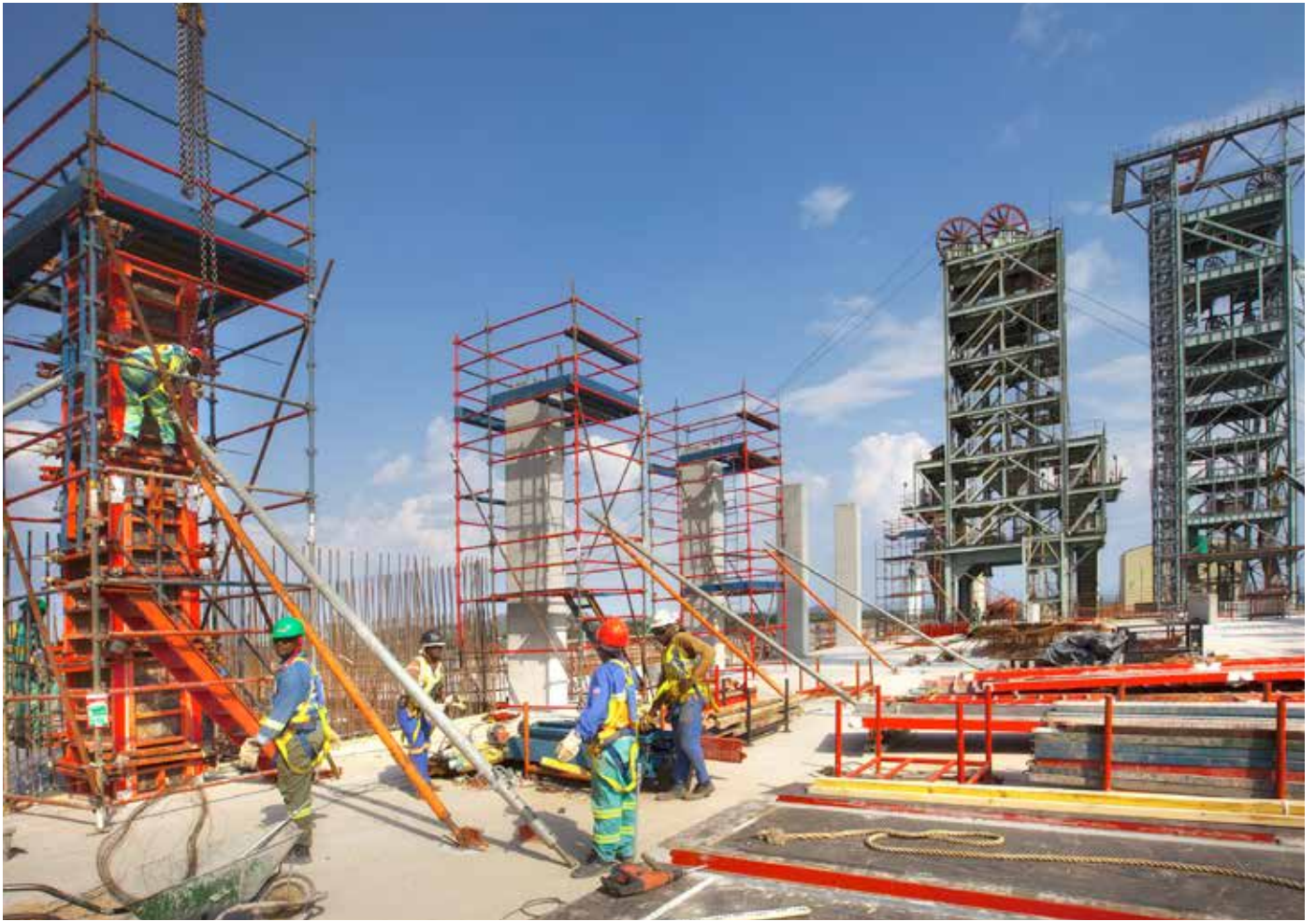
Construction at 17 Shaft, Impala
