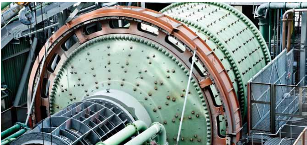
Primary ball mill undergoing routine maintenance
