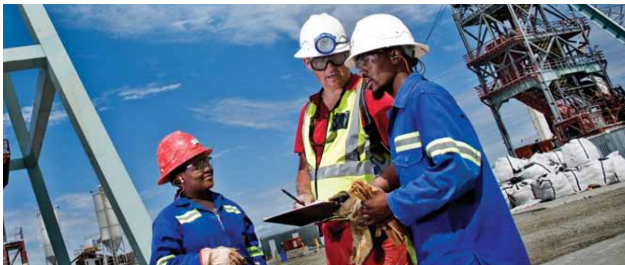
Styldrift I Project under construction
