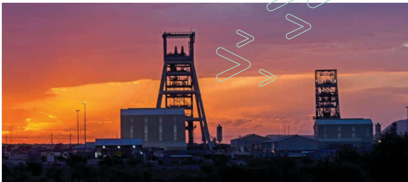
Main and Services shaft headgear at Styldrift I
