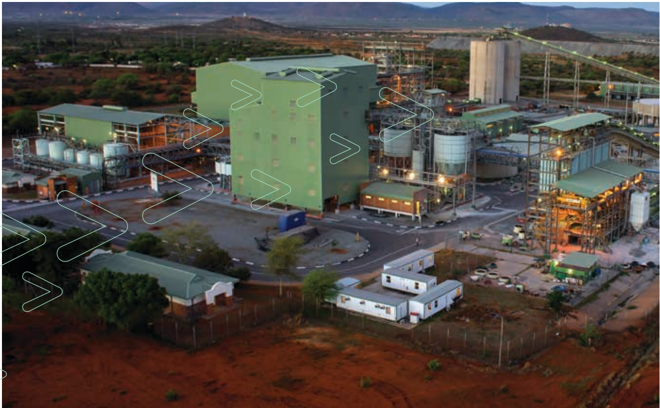
BRPM concentrator plant
