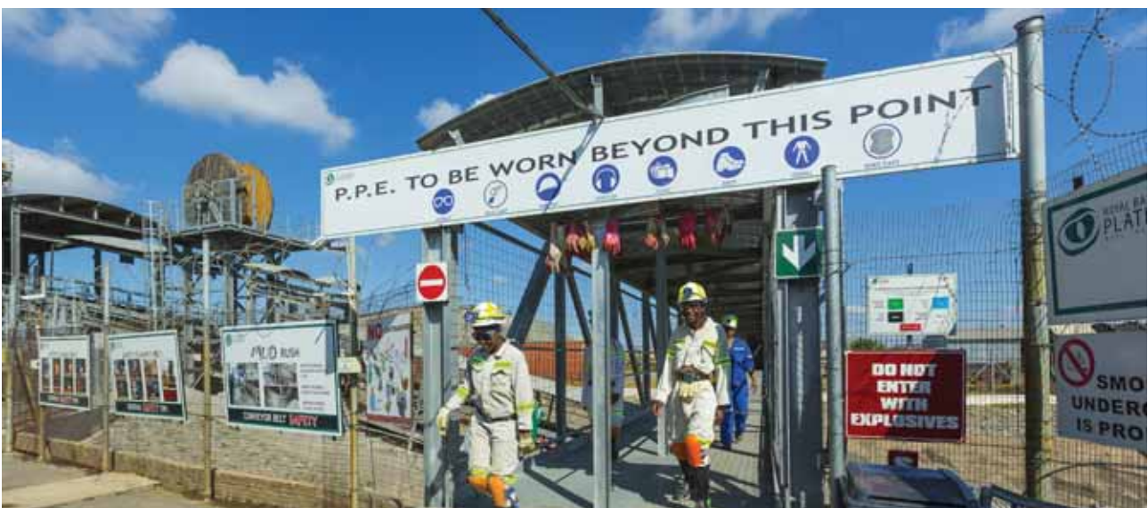
Entrance to BRPM North shaft portal area
