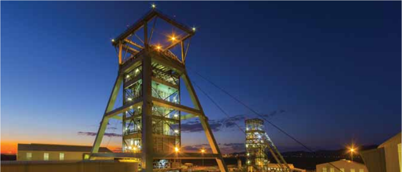
Main and Services shaft headgear at Styldrift I
