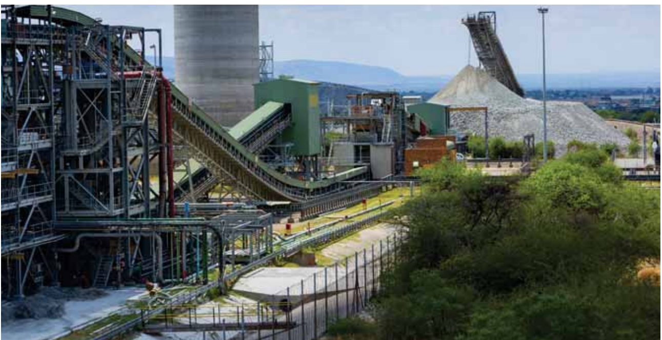
BRPM concentrator plant and run of mine stockpile
