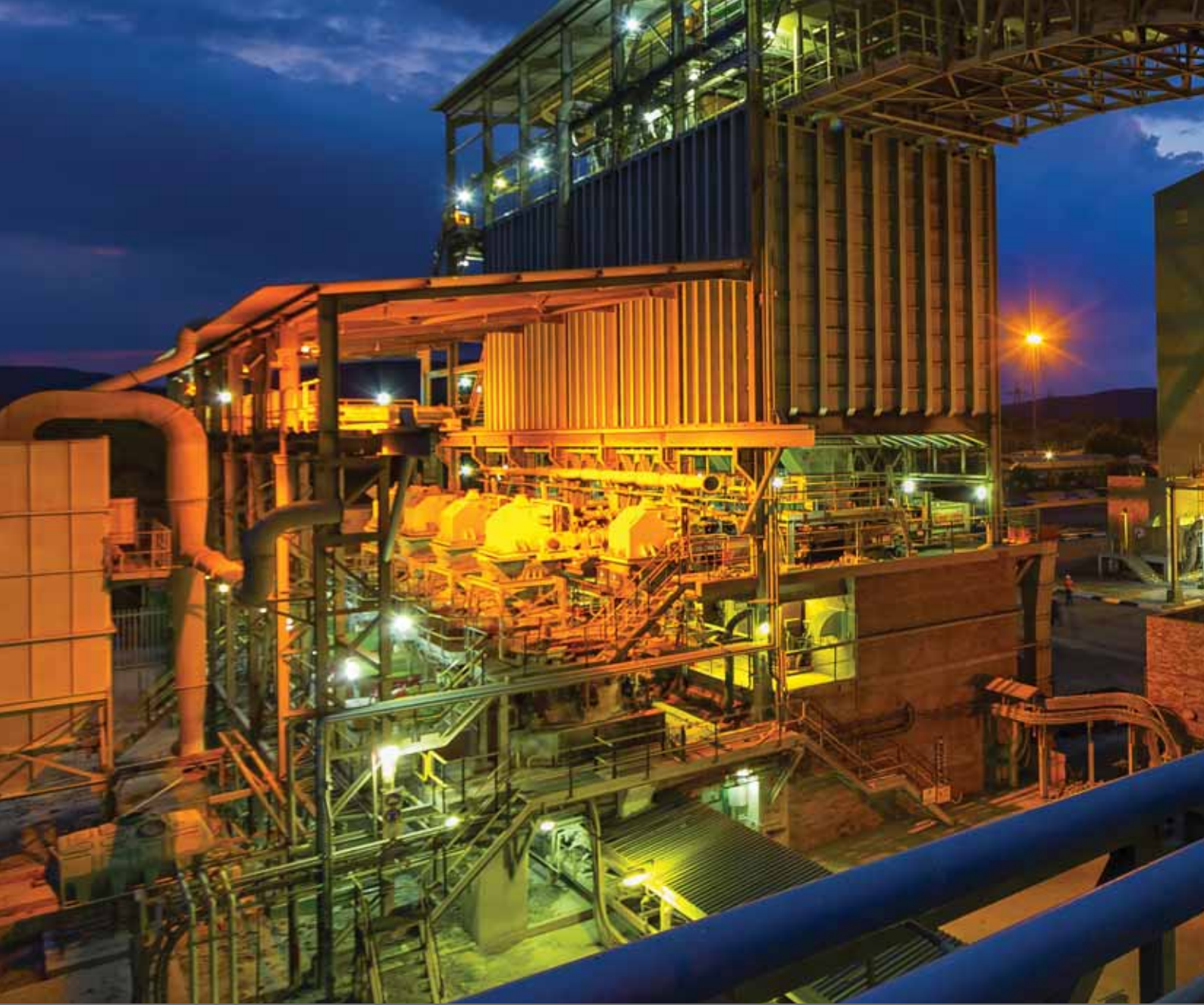
BRPM concentrator plant
