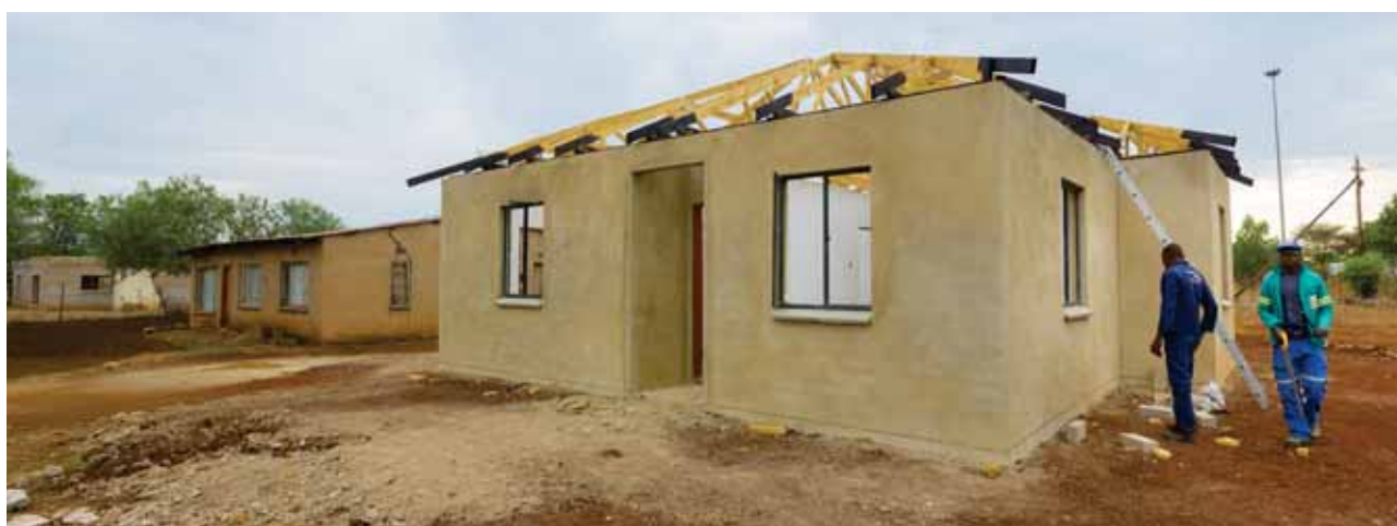
We constructed 19 new houses in MACHARORA to replace unsafe houses
