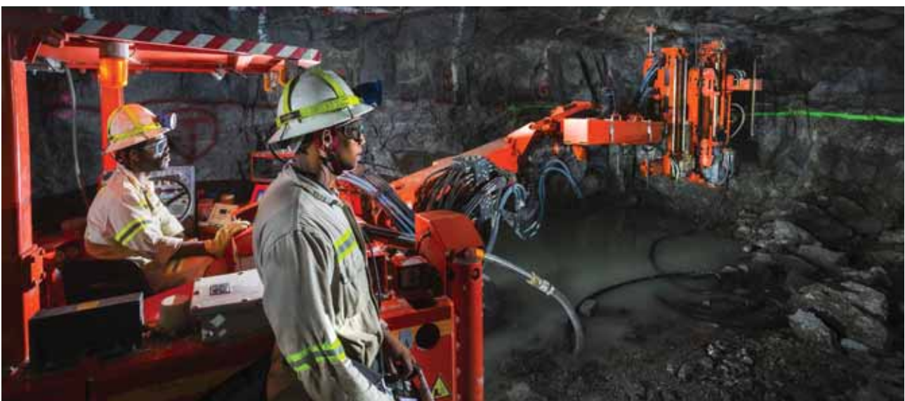
Mechanised bolter installing support at our Styl drift I project
