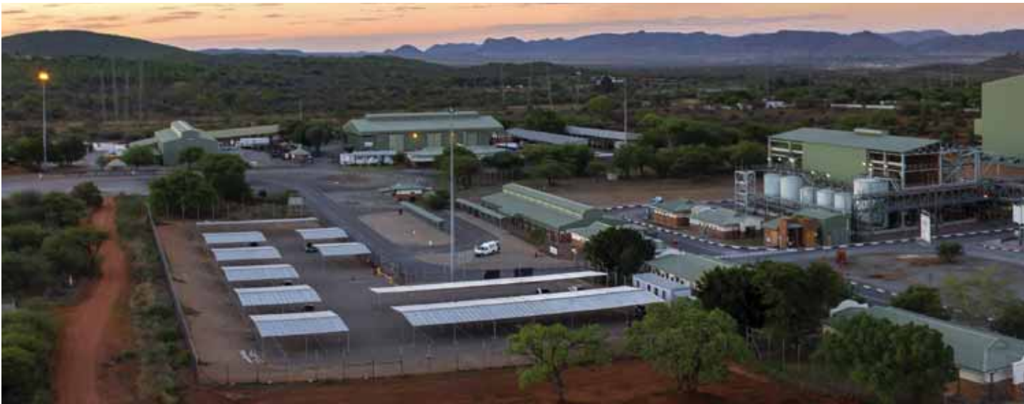
Our BRPM concentrator plant
