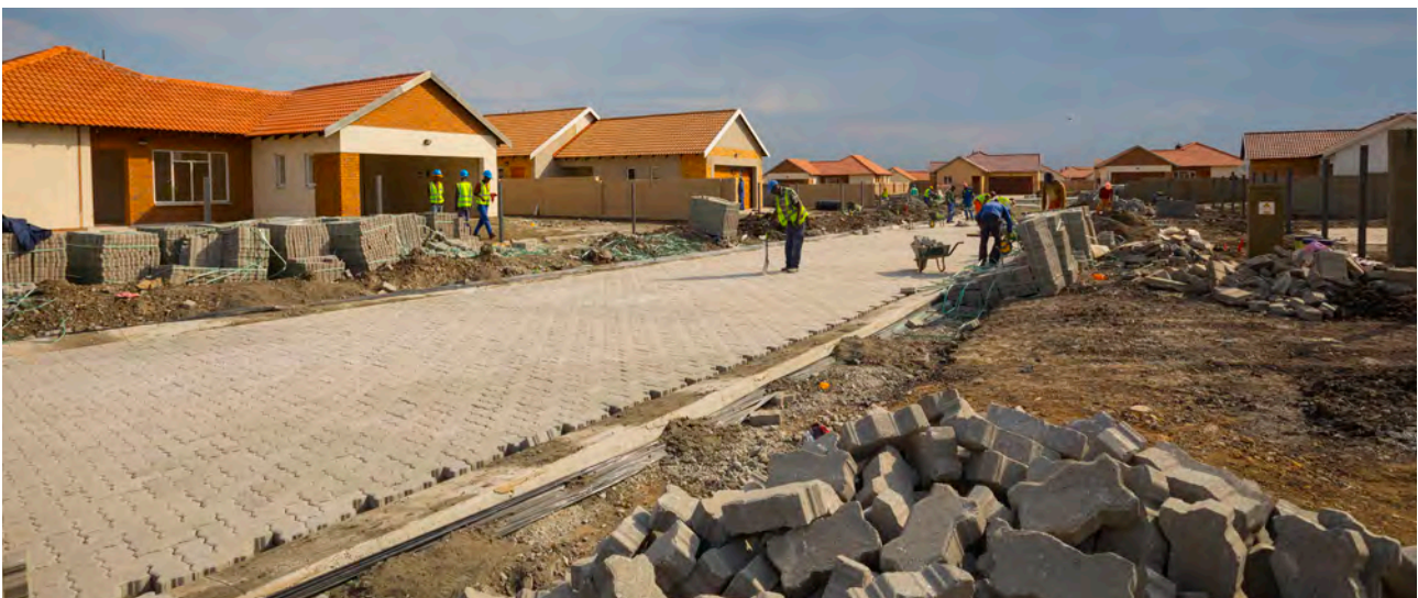
Phase 2 of our home ownership scheme under construction
