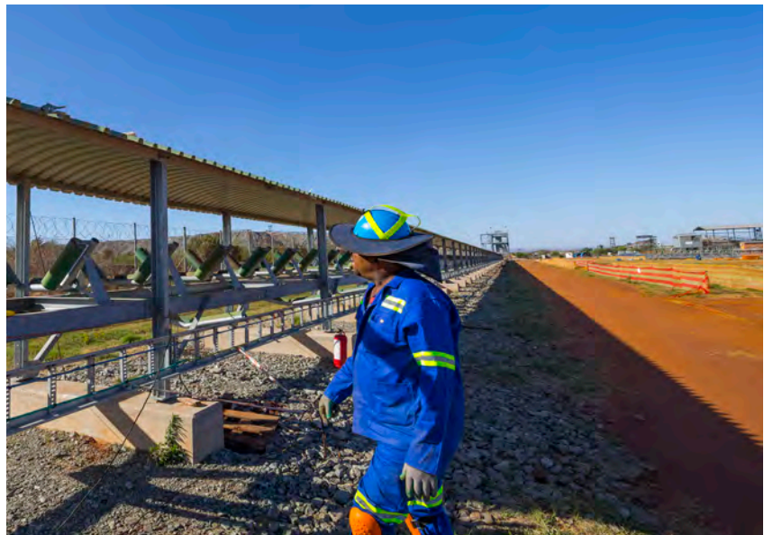
Conveyor belt between Styldrift I and BRPM concentrator under construction
