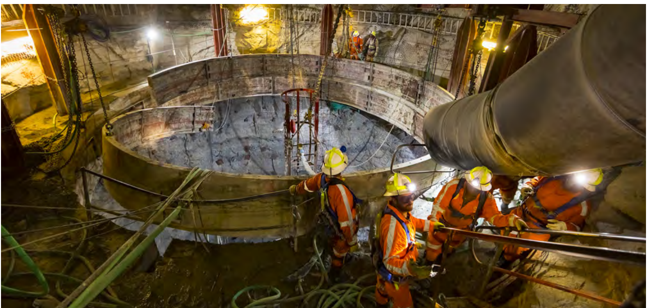
Settler 1 clarifier collar construction
