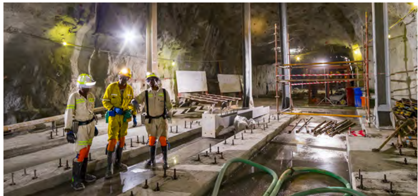
Silo 3 bulkhead construction
