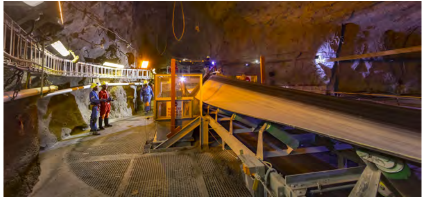
Ore pass discharge on 642 level
