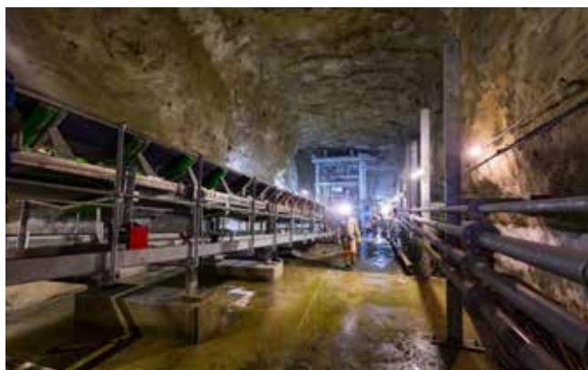
642 level North decline conveyor
