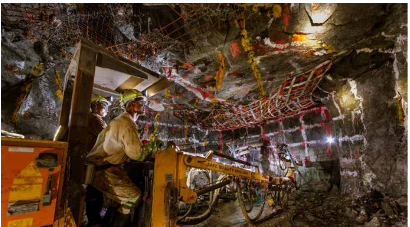
Strike drive development drill rig in the hybrid mining section on 14 level at BRPM
