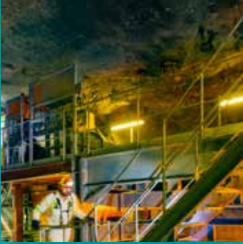
South dip conveyor in bulkhead installation on 642 level
