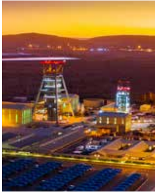
Solar-powered street lights at Styldrift Mine
