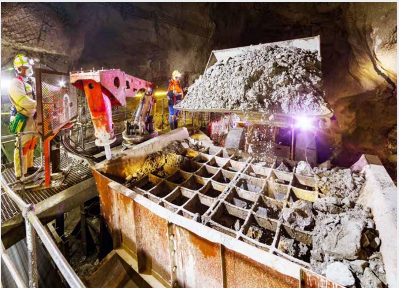
Tipping of ore in Phase III 114 level hybrid mining section at BRPM
