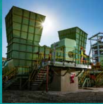
Vent shaft No 3
