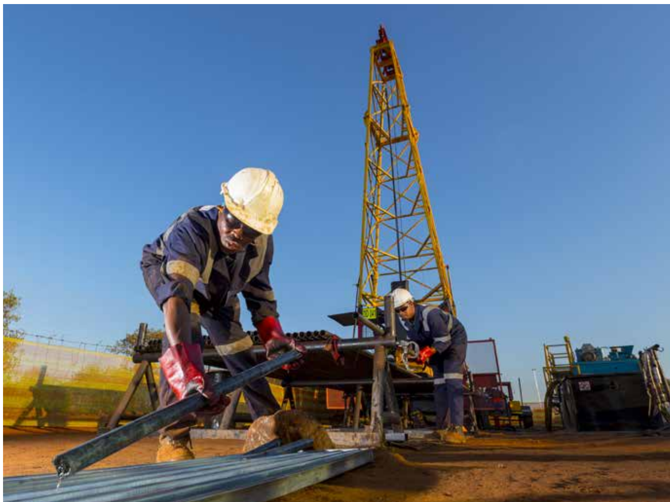
Exploration drilling operation, BRPM North shaft Phase III
