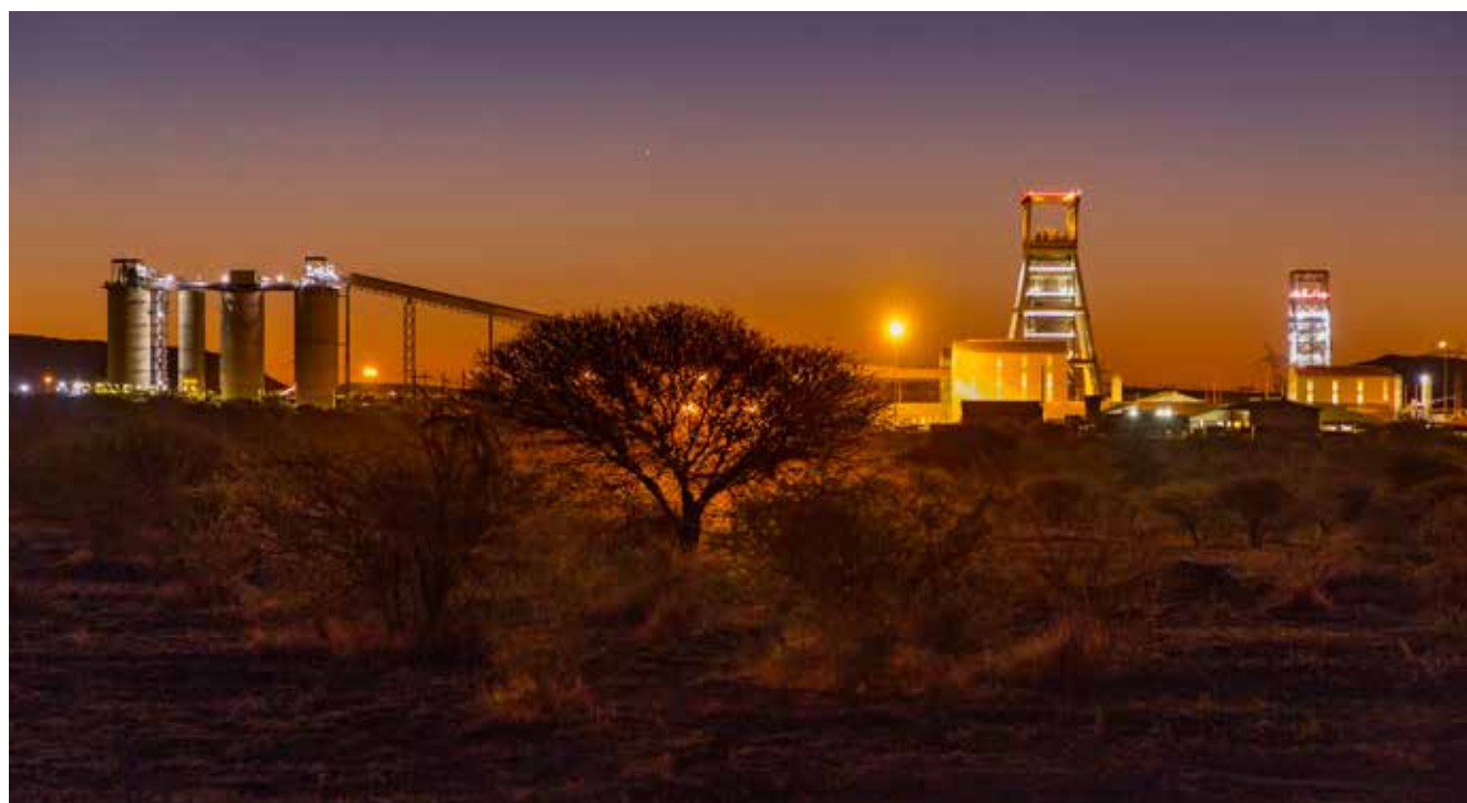
Styldrift I Main and Services shaft
