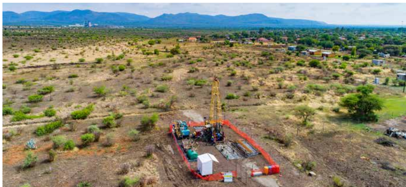
Exploration drilling operation, BRPM Phase III
