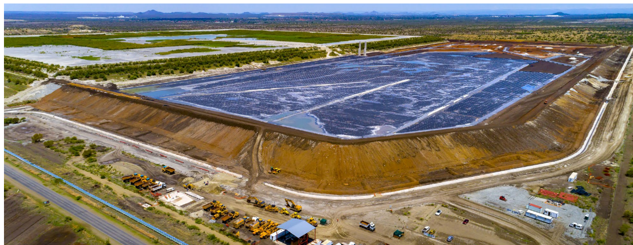
The extension of the current tailings facility at BRPM
