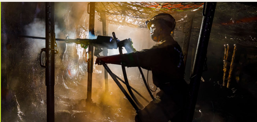
Rock drilling at BRPM
