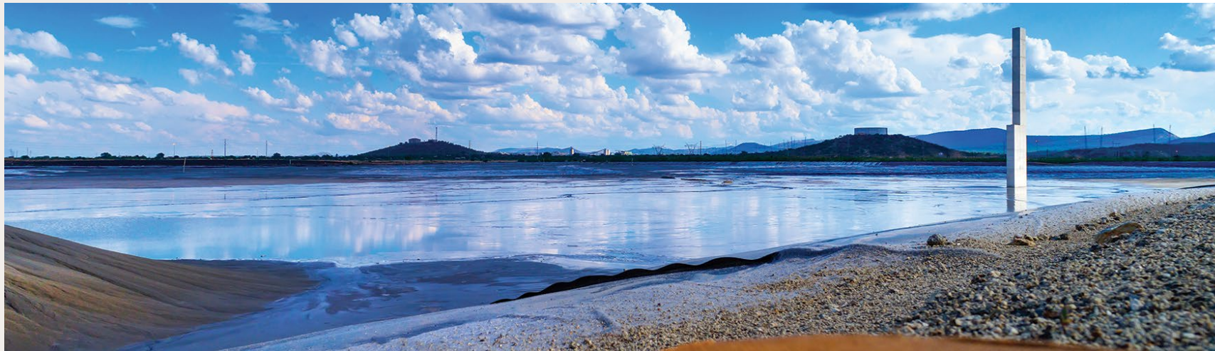
The upgrading of the Maseve tailings storage facility
