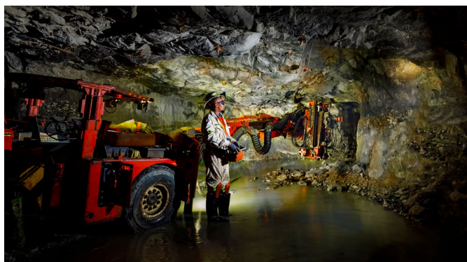
Mechanised roof bolt installation on 600 Level at StylDrift
