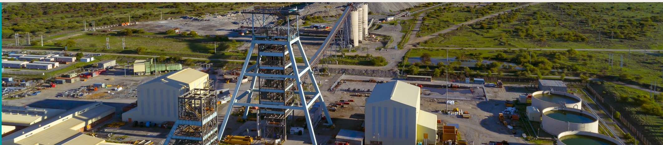
View of Styldrift Main shaft and silo feed conveyor, as well as rock and main winder houses
