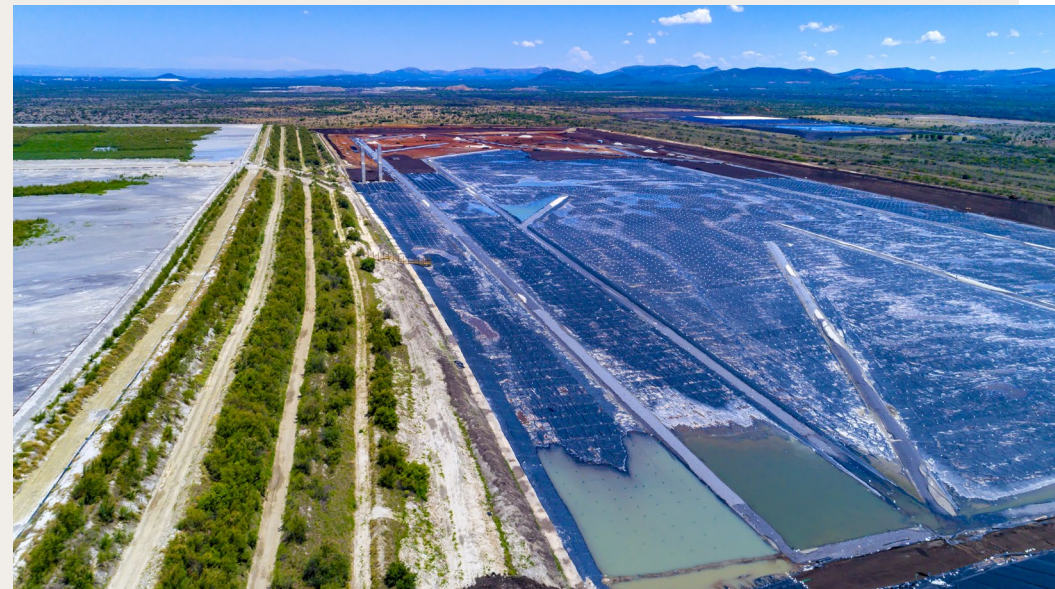
A view of the BRPM TSF upgrade
