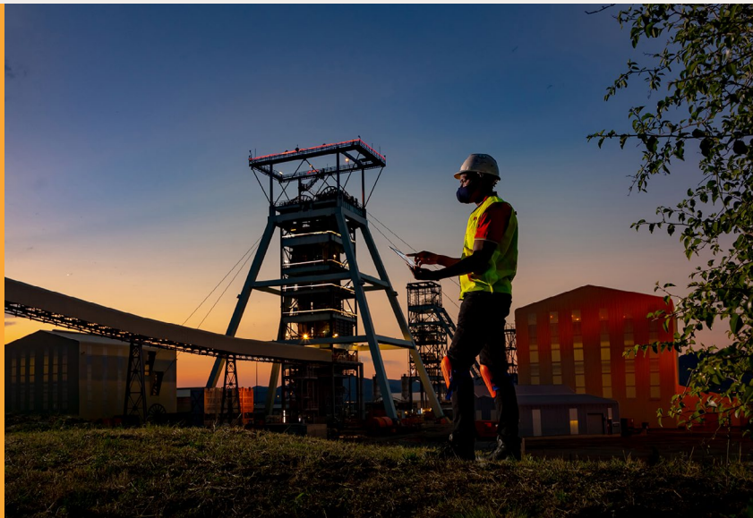
A view of Styldrift Main and Services shafts
