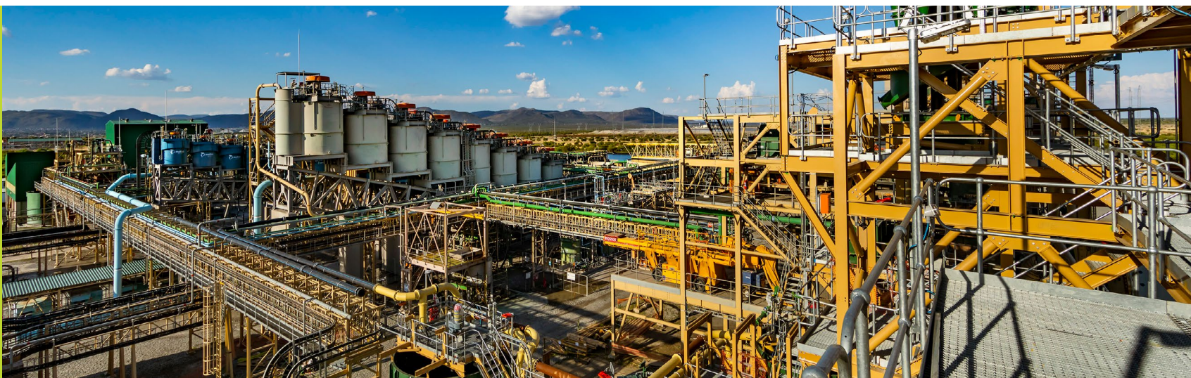
The MF2 upgrade at the Maseve concentrator under construction
