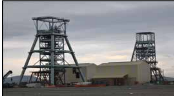
Main and services shaft headgears
