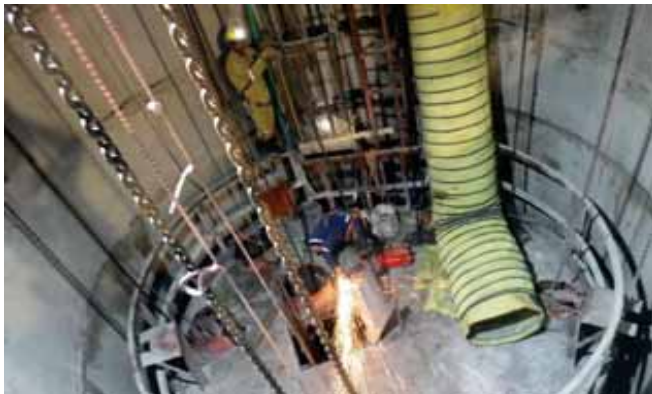
642 level - view of Settler 1 construction
