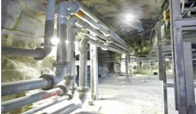
600 level - Permanent piping installation
