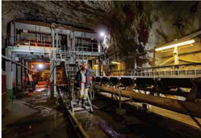
708 Level - Bulkhead No.3 and shaft loading box transfer belt
