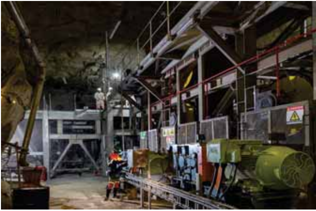
642 level - top of Silo 4
