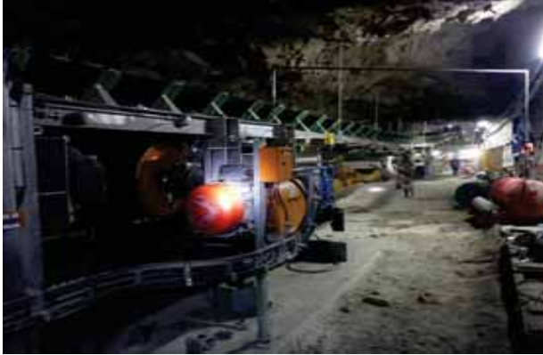
600 level - N1E Stope Conveyor installation
