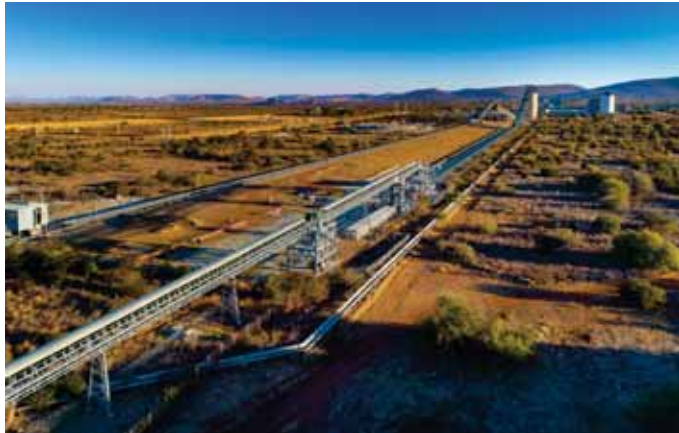
Styldrift overland belt to BRPM plant - 6.8km
