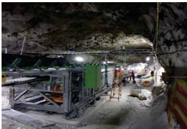
600 level - N1W Conveyor installation
