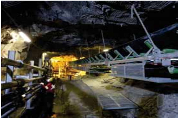
600 level - T03 transfer conveyor
