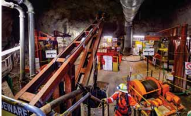
642 level - top of Settler 1
