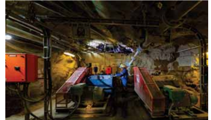
708 level - SP200 Dam and pump station
