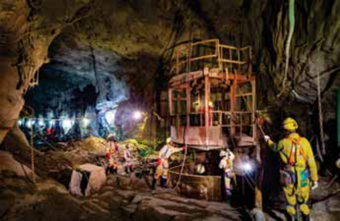
642 level - top of Silo 3
