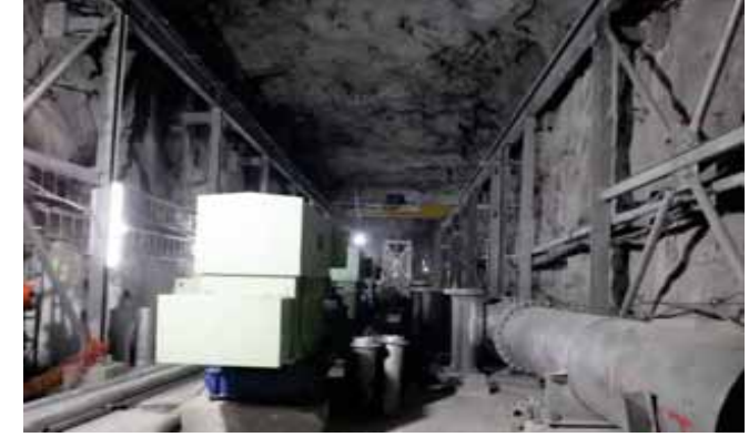
708 level - MPS piping under construction
