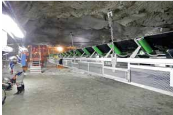
600 level - N2W Conveyor installation
