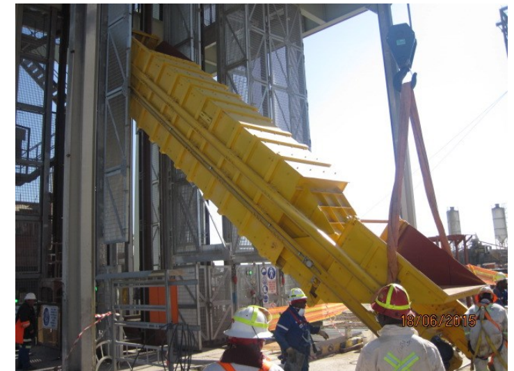
Styldrift Main shaft – 22 tonne skip being installed
